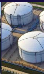
Oil Storage Tanks
